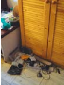
Loose wires on floor
