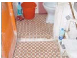
Same pattern of flooring and kerb
